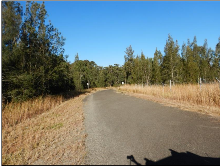
Figure 9: Sealed access road to existing spillway at approximately Ch 3120
