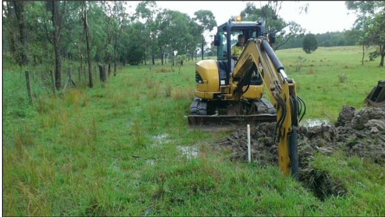
Figure 13: Ponded water near Pit 203 excavated during previous investigation (December 2014)
