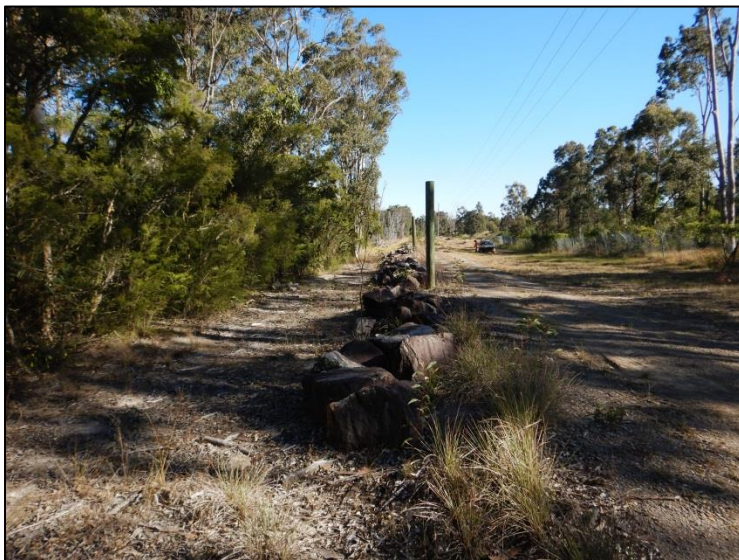
Figure 6: View of start of existing access embankment, looking south-west
