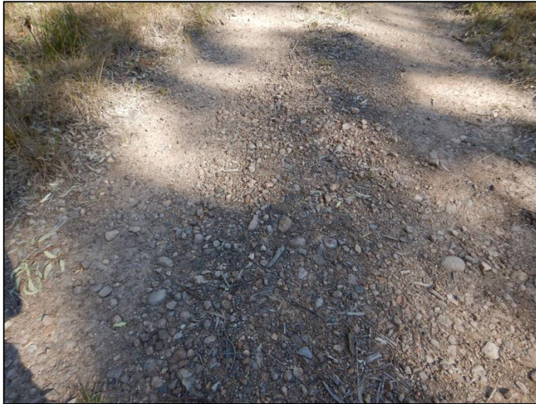
Figure 19: Typical gravel placed along access tracks
